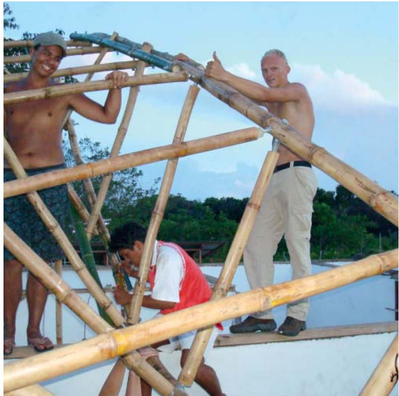
Bamboebouwwerk in Suriname (Credit: Foto: Reshmi Oemrawsingh).
